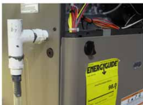
Figure 4: External Short Drain Tee
